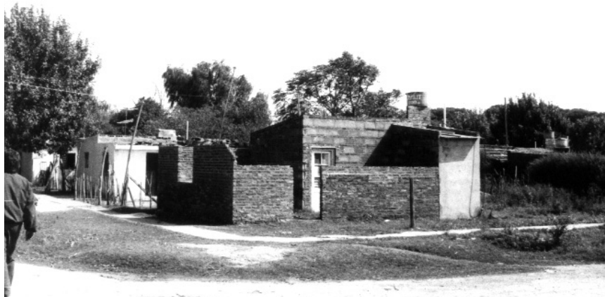
above Basic unit enlarged by a bathroom; further rooms under construction Sta. Fé, Argentina
